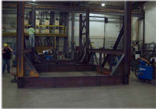
Preassembled load Out Structure
